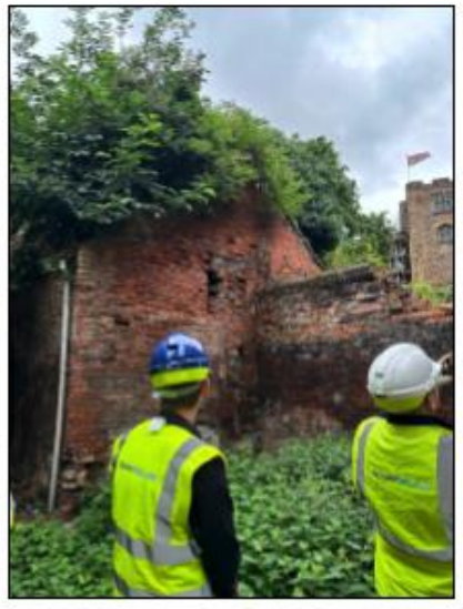
Photo A Existing outbuilding and castle wall
