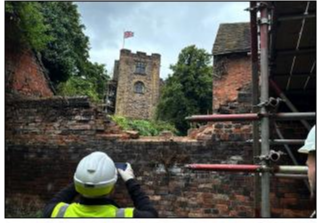
Photo C Existing outbuildings and garden wall with castle wall behind
